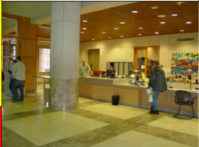
Another job well done – recently completed circulation desk project at the second floor entrance of Hodges Library.
