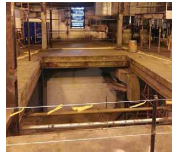
Removal of Boiler #1
