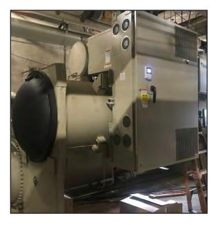
Pictured to the left is the new Daikin chiller installed by the A/C and Plumbing Services teams in the Andy Holt Chiller House. Another new chiller will be installed at the other end of the chiller house to serve the Communications building.
