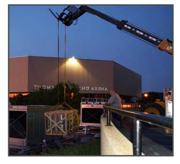
The new fan units will work to remove any heat that the equipment in the machine room puts off and vents any fumes that may be coming from the equipment or equipment repair. The old fans were over 30 years old and were worn out.
