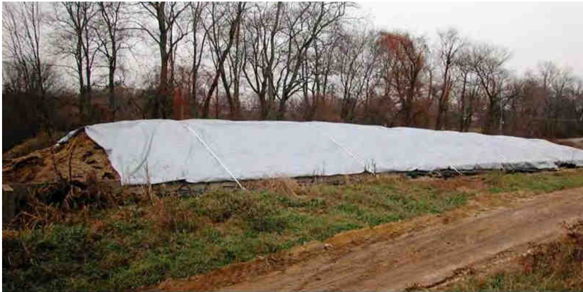
Temporary covering was used to protect the topsoil stockpile from erosion.
