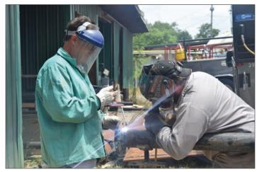
Exploratory dig and repair as needed on steam line at Ellington Plant Science.
