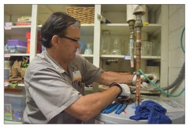
Installed 5 new 6" water valves at steam plant on the water station.
