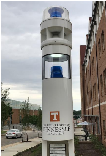
Typical Code Blue Phone on a Pedestal
