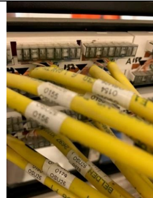
Sample Rear of Patch Panel Labeling
