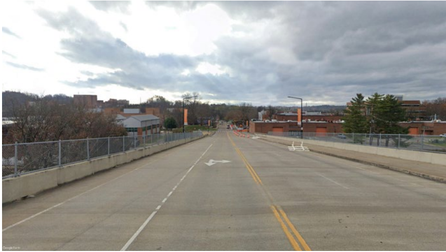
Joe Johnson Drive - Existing
