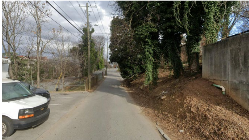
Caledonia Avenue - Before
